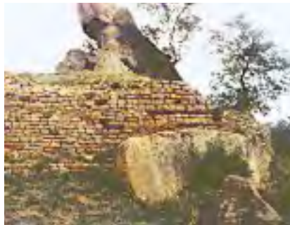
A workshop on Dry Stone Masonry (see box, page 23) was held at the World Heritage Site of Great Zimbabwe, once an important trading centre. Its intricate complex of dry stone walls, extending over nearly 80 hectares, attests the Bantu civilization of the Shona people between the 11th and 15th centuries.
