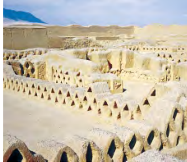
The World Heritage Site of Chan Chan, Peru, capital of the Chimu kingdom, which reached its peak in the 15th century. The adobe, or earthen, structures are endangered by natural erosion from rain and air.
