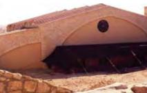
Enclosure over the Church of the Apostles, Madaba, Jordan. The western orientation of the facade and the use of glass resulted in damage to the mosaics from solar radiation, leading to the replacement of the glass with concrete and wooden panels.
