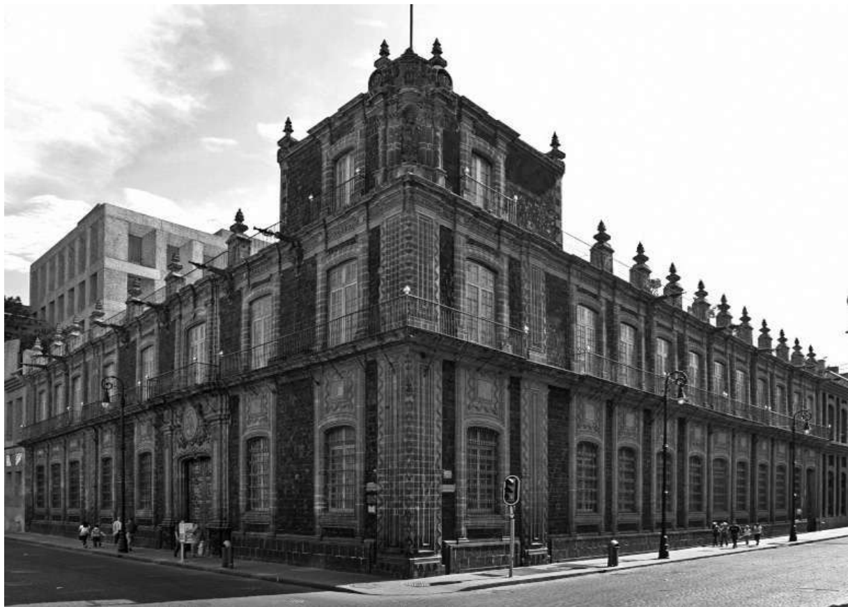
PALACE OF THE COUNTS SAN MATEO DE VALPARAISO, WITH THE FAÇADE COVERED WITH TEZONTLE STONE. Image: Public domain.
