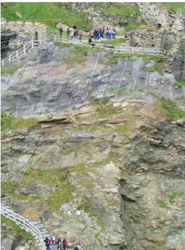
Fig. 5. Metal containment nets are one method employed to retain unstable rock slopes, as on this mediaeval site of Tintagel, England (©Arthur McCallum – English Heritage)
