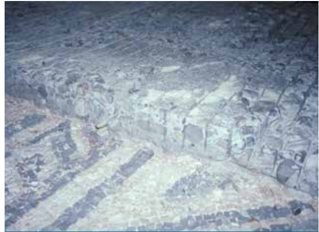
Fig. 12. Removal of cement mortar from the back of a pavement, by mechanical incisions, and working with a hammer and chisel
