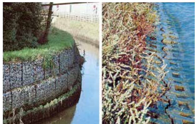
Fig. 7. Protection of an embankment with gabions (Maccaferri)
