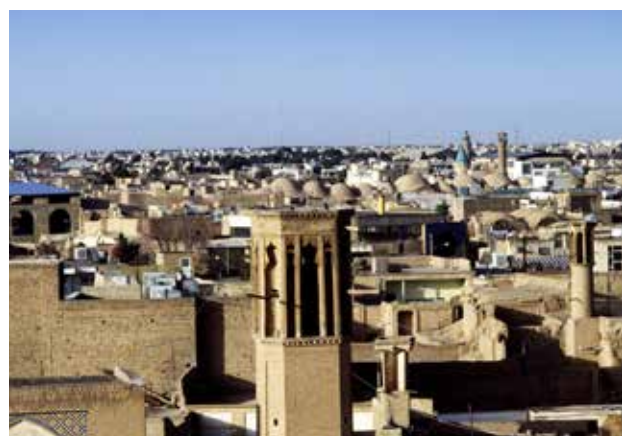
Fig. 5. Kashan. The historic city of Kashan, Iran, has retained much of its historic integrity, particularly that of its building fabric, and its wind-tower-based traditional ventilation system. In recent years, housing complexes have been rehabilitated as hotels. However, many of its fragile mud brick buildings risk decay and even collapse if not properly used and regularly maintained.
