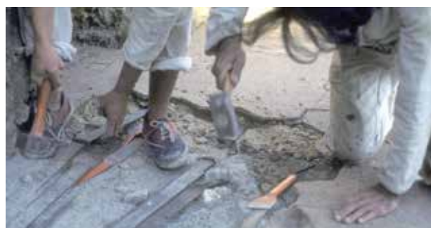
Fig. 11. Undercutting a pavement with iron bars, requiring great skill and judgement to prevent damage
