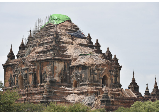
Figure 5. The Sulamani Temple, one of the oldest temples in Bagan, suffered extensive damage to its structure and interior objects due to the 2016 earthquake
