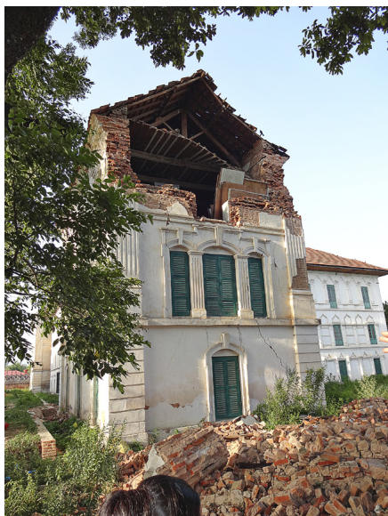
Figure 1. The oldest building of the National Museum of Nepal suffered extensive damage and contained a large collection that had to be evacuated
