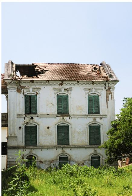
**Figure 1.** Main historical building of the National Museum, heavily damaged by the 2015 earthquake
