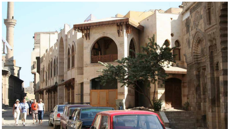
► Figure 4.43 A training centre built in 2008 with the use of historic architectural vocabulary
