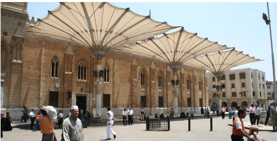
◀ Figure 4.45 High-tech shading devices manufactured in Germany that were designed for the Ministry of Awqaf by Egyptian architect Muhammad Kamal
