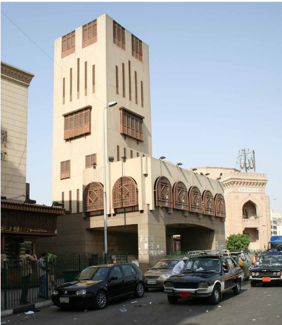
◀ Figure 4.38 A ventilating shaft of al-Azhar car tunnel
