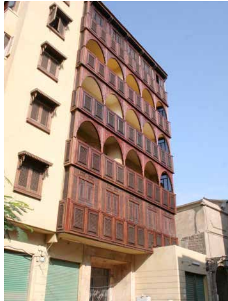
◀ Figure 4.37 A residential building constructed in the 1960s in al-Mu'izz Street. The façade was embellished with wooden lattice work and the building rehabilitated as a hotel
