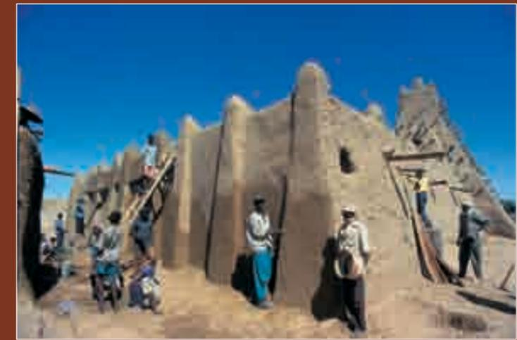
FIGURE 29 (top right) Replastering the western façade of the Sankore Mosque.
