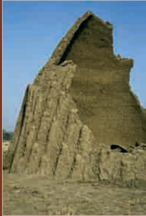
FIGURE 98 An abandoned hut reveals the slenderness of the casing.
