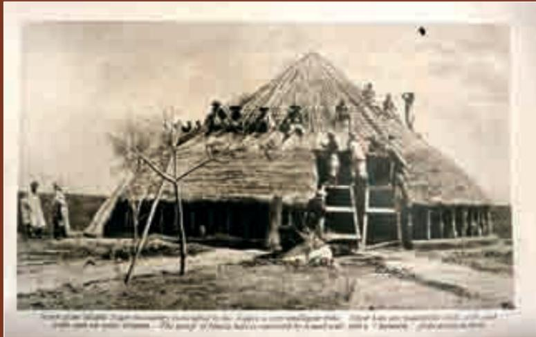
FIGURE 2 Communal work on the re-roofing of a ritual house, Nupe, Nigeria.
