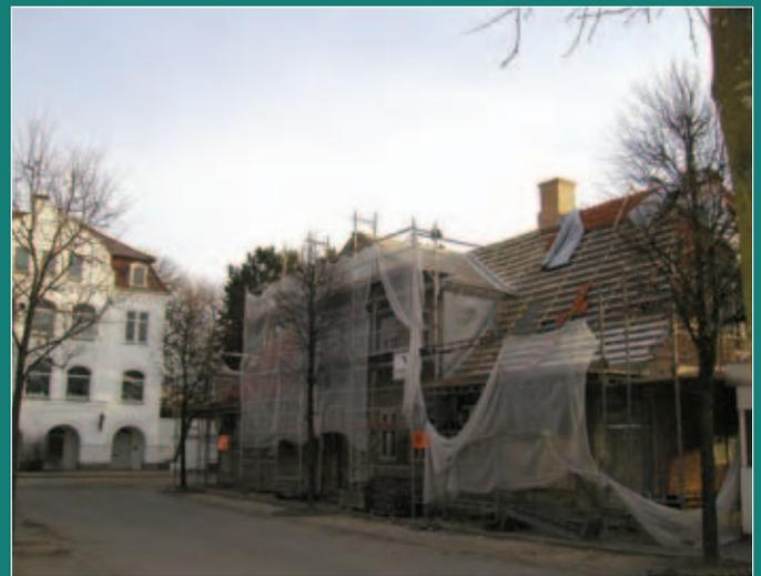
FIGURE 13 Restoration of Museumsgade No. 6. The roofing, windows and the wall exterior are being renovated.
