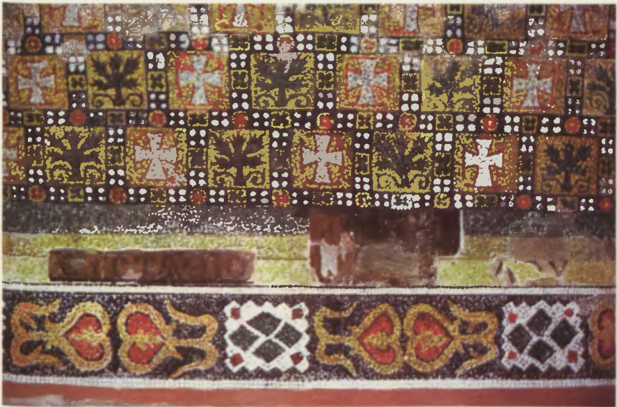
2. North side of the barrel vault. Detail of the modern intervention and of the earlier restoration.
