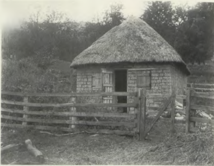
2. Protective structures over mosaics at Great Witcombe, Gloucestershire, erected 1819 and subsequently modified (© Crown copyright, NMR).
