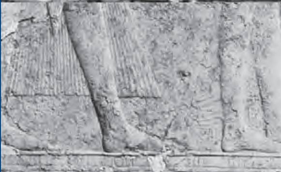
The same bas-relief 70 years after: damages caused by crystallization of salts.
