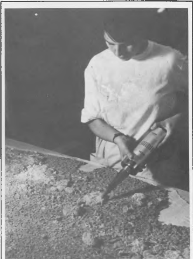
Fig. 6 - Cleaning of the tesserae with an ultrasonic hammer
