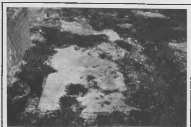
Fig. 3 - Partial infestation helped by calcination and sinking
