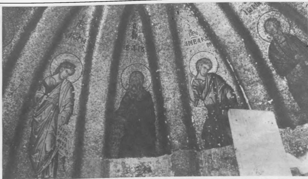
Fig. 6 - Dome of the Fethiye Djami in Istanbul during conservation. Covering plaster has been removed from the lower part of the mosaic and cramps have been used to reattach the mosaic to the masonry
