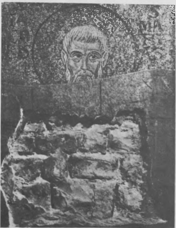
Fig. 4 - The stones of the wall itself are revealed when all the mortar has been removed
