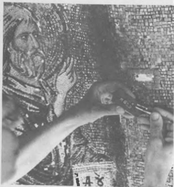
Fig. 12 - Replacing the cubes that had been removed for installation of the cramp
