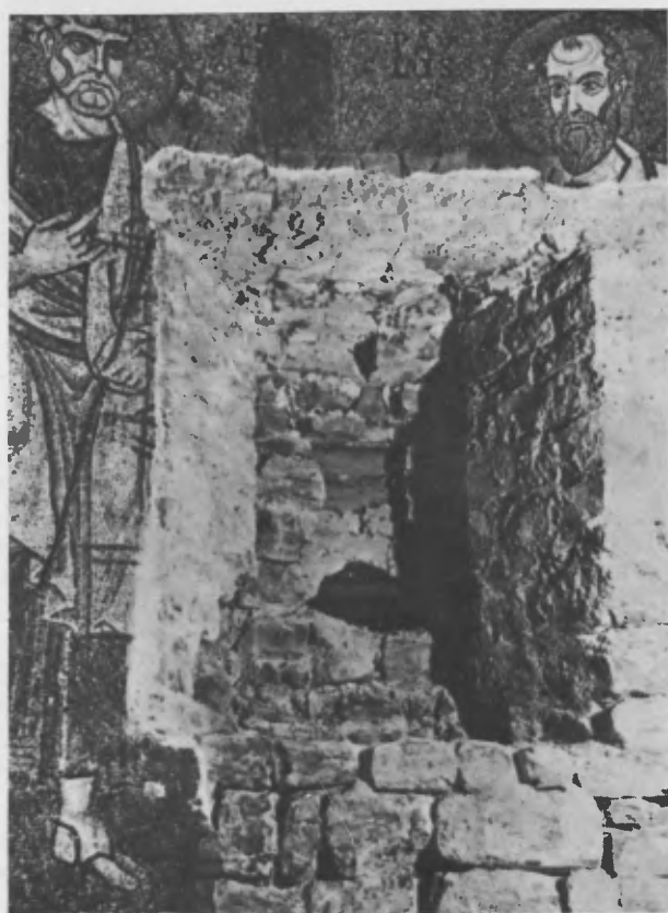
Fig. 8 - The removal of the mosaics, successive layers of mortar, and the cleaning of the underlying masonry, brought to light a series of windows which existed before the present mosaic decoration of the apse
