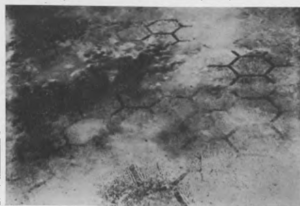
Fig. 9 - Development of algae on a mosaic in a damp and poorly-lighted place
