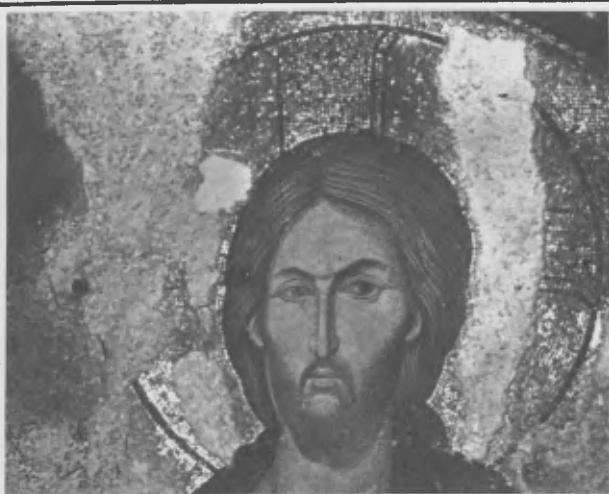
Fig. 14 - Detail of the Deisis mosaic of the Kariye Djami, Istanbul, during cleaning and consolidation. A new inscription has been found in the painted plaster where cubes have fallen. Holes have been filled with lime plaster
