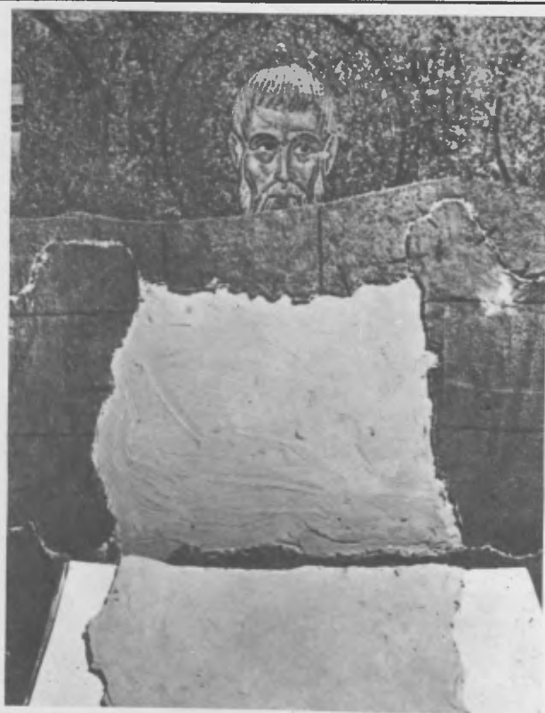
Fig. 5 - The new mortar bed is ready to receive the mosaic
