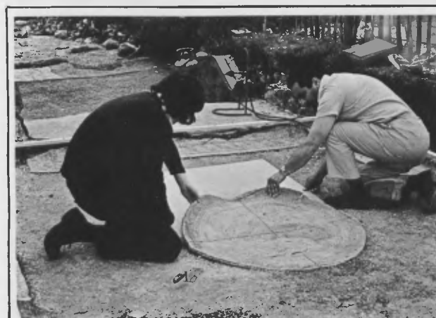
Fig. 7 - Hare Pavement, Cirencester Central motif section being slid carefully onto panel board for safe handling, reversing and cleaning. Note grid lines in both directions.
