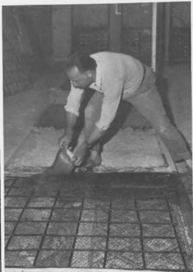
Fig. 3 - A cement mortar is applied over the metal framework attached to the back of the mosaic
