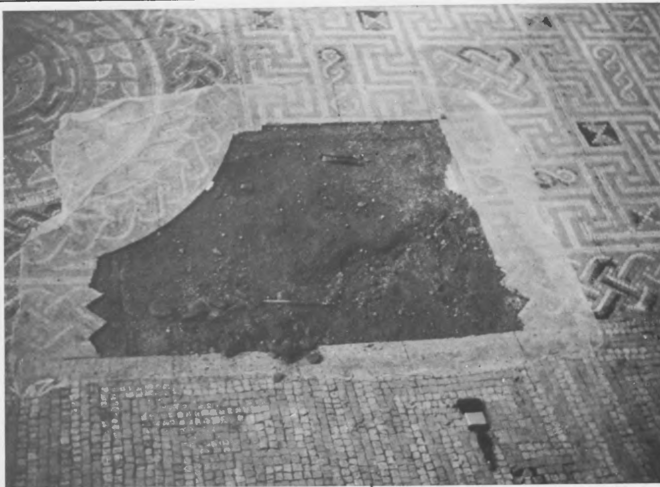
Fig. 8 - The Great Pavement, Woodchester. The surface has been covered with scrim following the pattern lines. A section has been cut out and lifted. The nucleus has been detached, disclosing a fracture in the base
