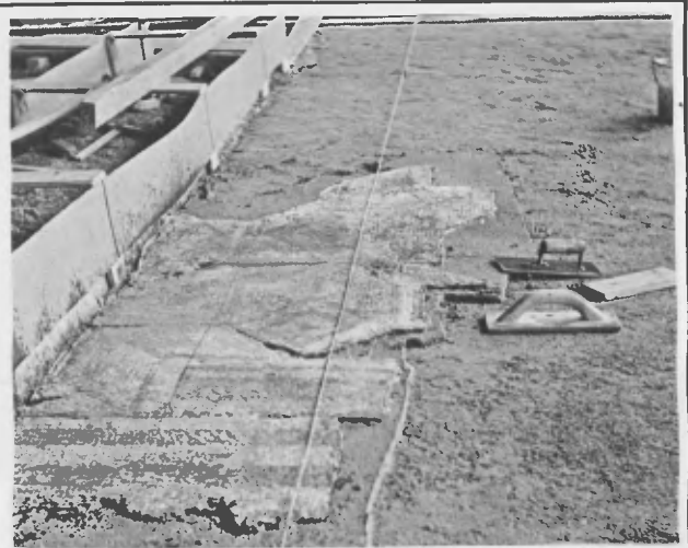
Fig. 2 - Roman palace, Fishbourne Geometric patterned mosaic being relaid. Note the grid lines being located to line across pavement from surrounding reference battens
