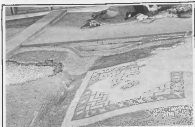
Fig. 8 - The lacuna is filled with pebbles
