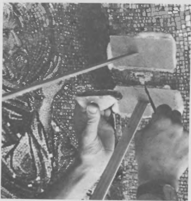
Fig. 11 - Plastering in the cramp in a wall mosaic. Braces are applying light pressure to the mosaic in an area where thinned lime plaster has been injected
