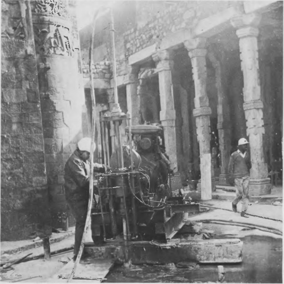
Fig. 9 - The Qutb Minar: Grouting holes around the Minar
