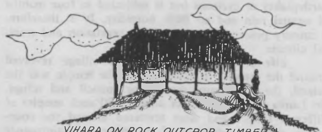
VIHARA ON ROCK OUTCROP, TIMBER FRAMED STRUCTURE INDEPENDENT OF WALLS. SHRINE IN MUD. TILE ROOF.
