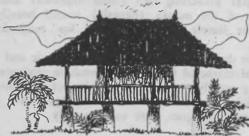
TAMPITA VIHARA - ON STONE PILLARS. TIMBER FRAMED. MUD WALLED SHRINE IN CENTRE. TILE ROOF.
