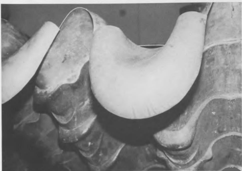
Fig. 8. Szymanów. Reconstruction of the lips of the fountain. After all the pieces were properly assembled, they were joined together by means of tin/lead solder.
