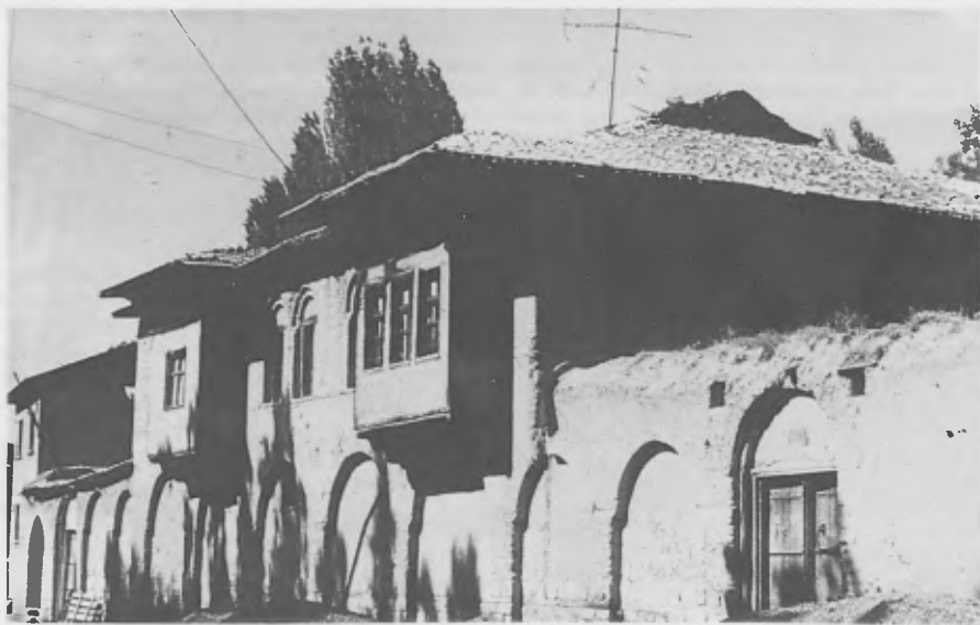
PIC.No.4. An example of a house in which the massive adobe and timber frame system used together.Old Malatya.
