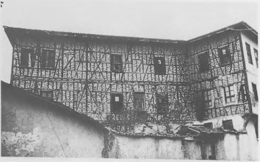
PIC.No.5 . An example of a house in which adobe blocks are used in between the wooden frame. Osmaneli, a small town of Bilecik.
