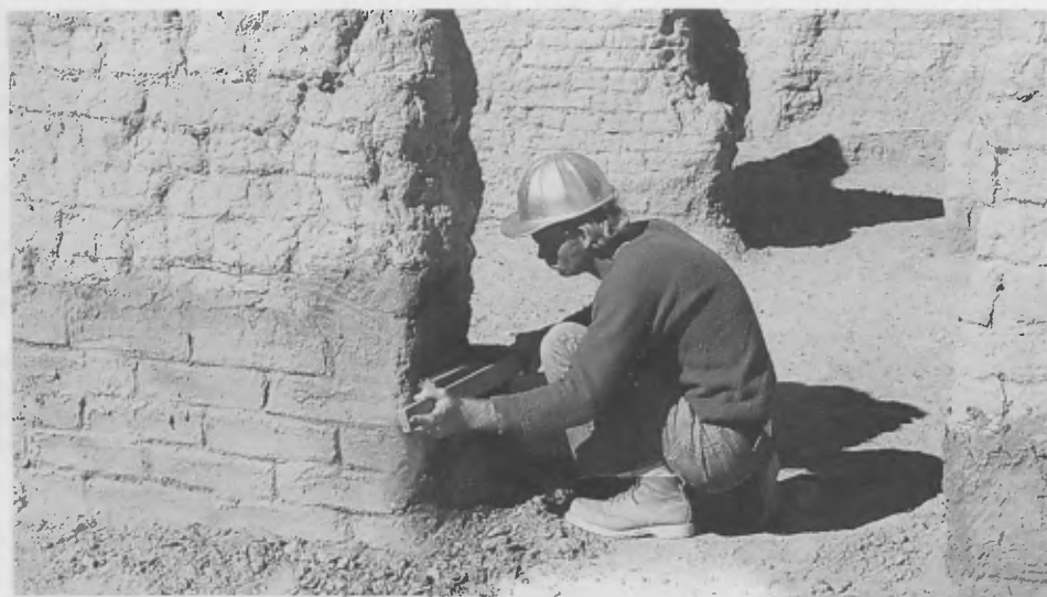
FIG. NO. 3 Wall base after correcting basal erosion with mud brick infill. Workman is filing down new brick to conform to historic wall profile.
