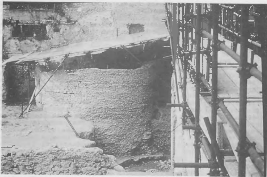
General view of the wall during excavation. The structure is already protected from rainwater and sun.
