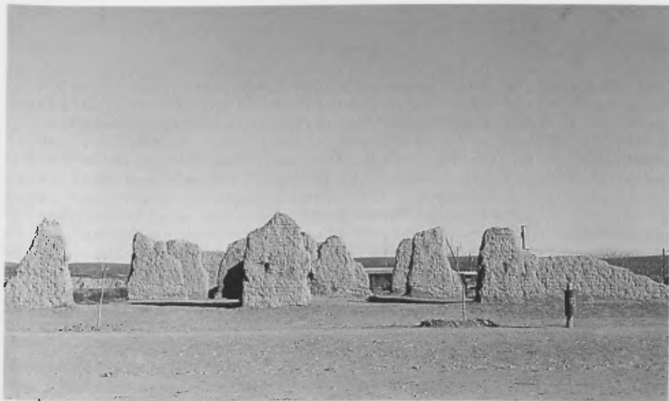
FIG. NO. 8 Officer's Quarters after stabilization in 1974. Note brick infill at base of walls and establishment of positive grade away from walls.
