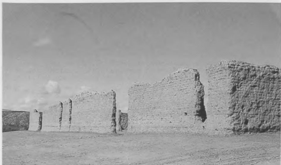
FIG. NO. 5 Company Quarters after stabilization. Note higher fill level and establishment of positive slope away from walls.
