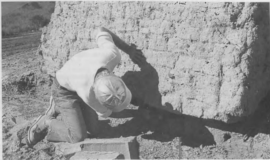
FIG. NO. 2 Preparing wall base for insertion of mud brick infill to repair damage caused by basal coving.
