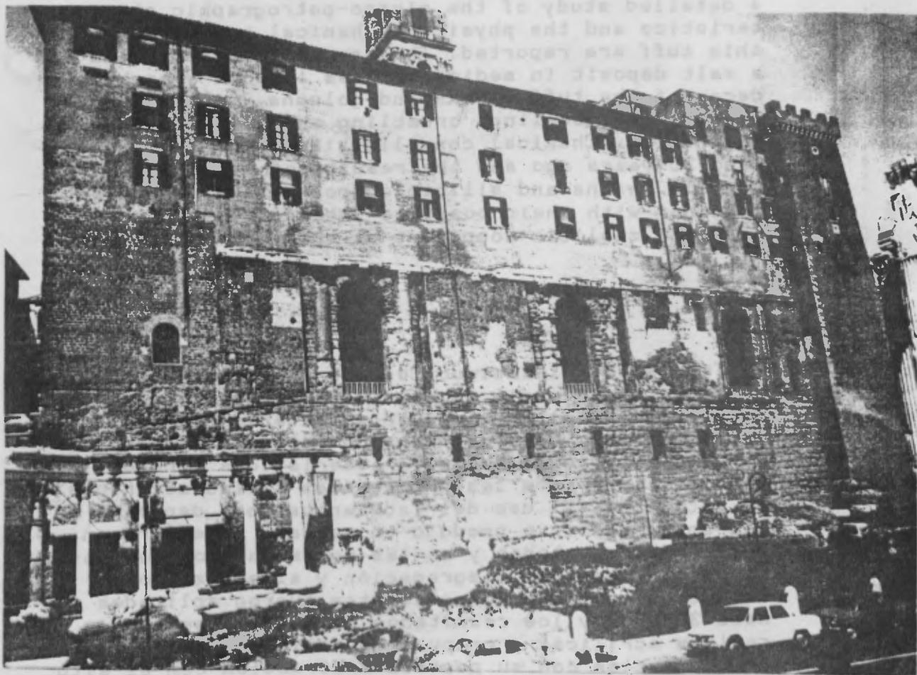
Fig. 1 - The structure of the Tabularium is located at the base of the Capitolium and overlooks the Roman Forum. In the lower part, there may be seen the lines of blocks of the Lapis Gabinus tuff, which also constitutes the columns bordering the entrances at half height. In the last few years excavations considerably lowered the field level and exposed the base of the wall.
