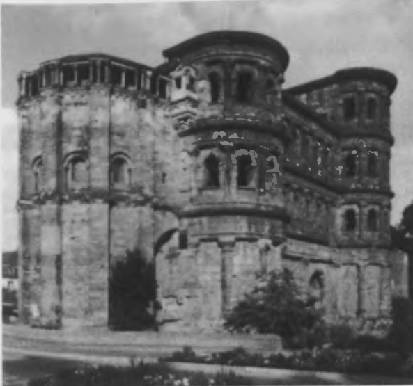
Fig. 1: Porta Nigra in Trier, roman construction
