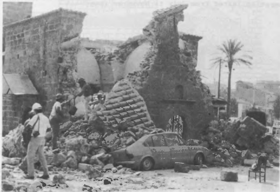
Fig 2. After the earthquake.
