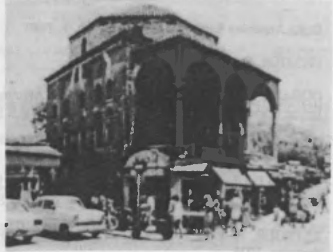
ATHENS, GREECE: Church reinforced with cables.
