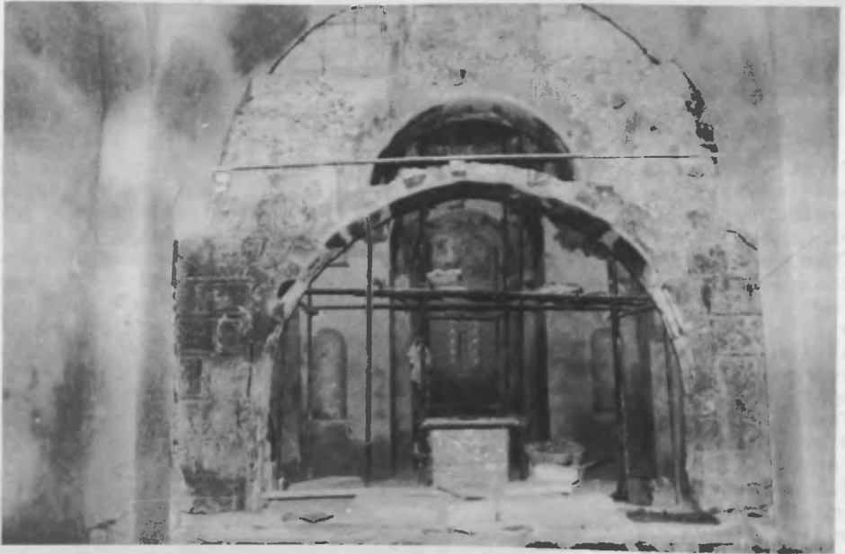
Fig 10. Interior view of the western arch.
