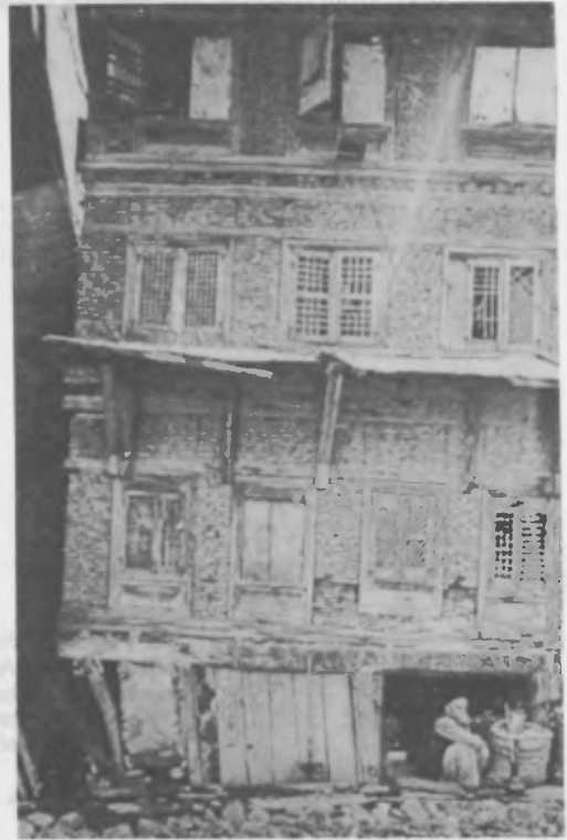
SRINAGAR, KASHMIR: A building designed for seismic resistance! An example of late 18th or early 19th century Taq construction.
