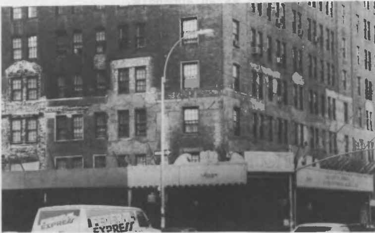
Figure 1. Overall view and details of the Mayflower Hotel, New York City, showing non-structural architectural decoration stripped in response to Local Law 10. Photo courtesy of the New York Times.
