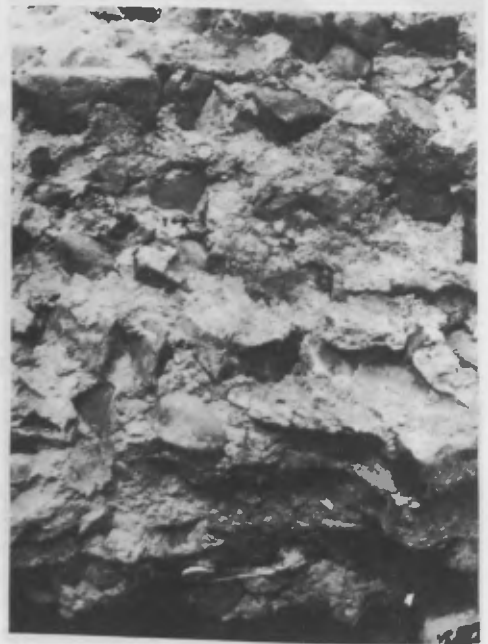
Figure 6: Corner section of wall showing brickwork skin Figure 7: Conglomerate inner section of wall
