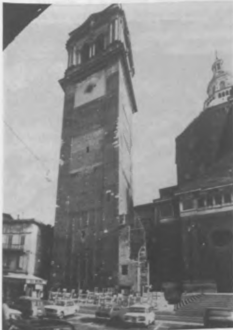
Figure 2: The Civic Tower and the Cathedral before collapse
