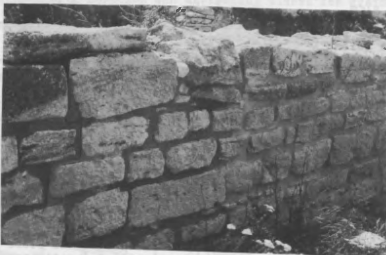
Photo No. 2 - Hydrophobically and non-hydrophobically treated part of the wall after rainfall
