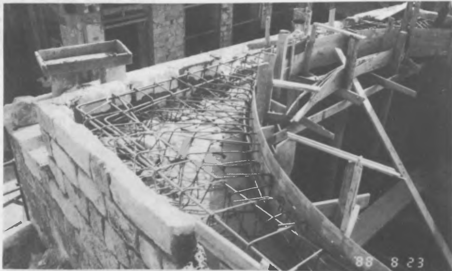
Fig 7. Reinforced concrete beam on the pendentives.
