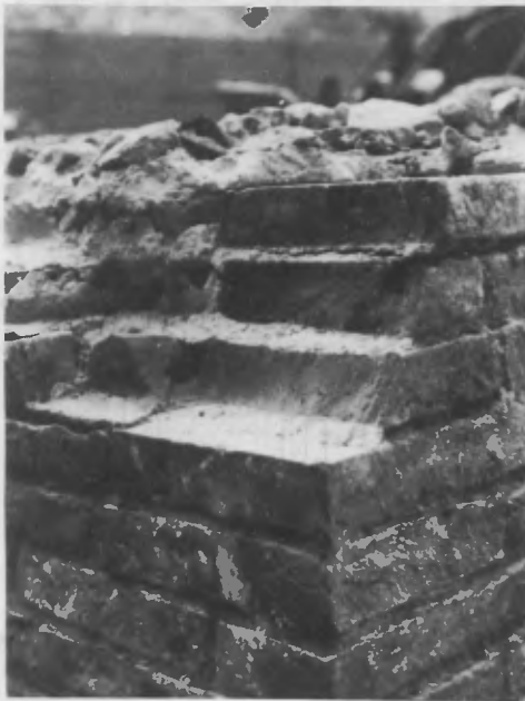
Figure 6: Corner section of wall showing brickwork skin Figure 7: Conglomerate inner section of wall
