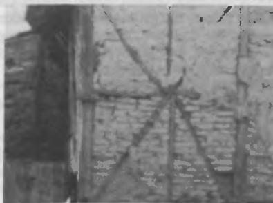
SKOPJE, YUGOSLAVIA: Brick nogged construction.
