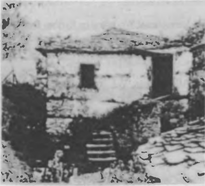
PELION, GREECE: Traditional stone house showing use of horizontal runner beams in stone walls similar to Taq.
