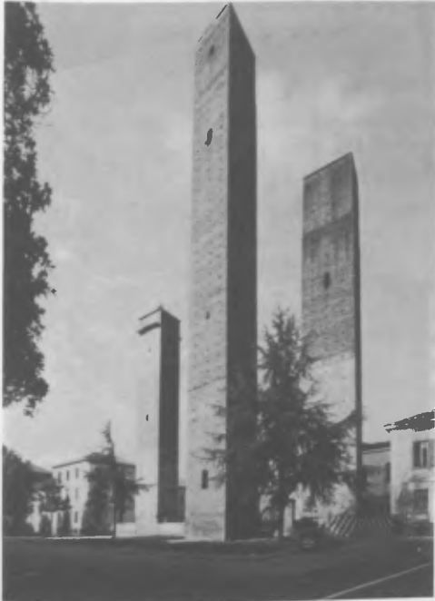
Figure 1: Medieval Towers in the historical centre of Pavia
