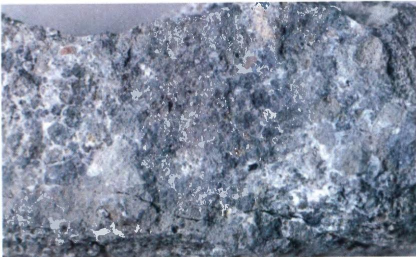
Figure 7.3 Typical surface of a Tabularium block, with exfoliation and scaling.
