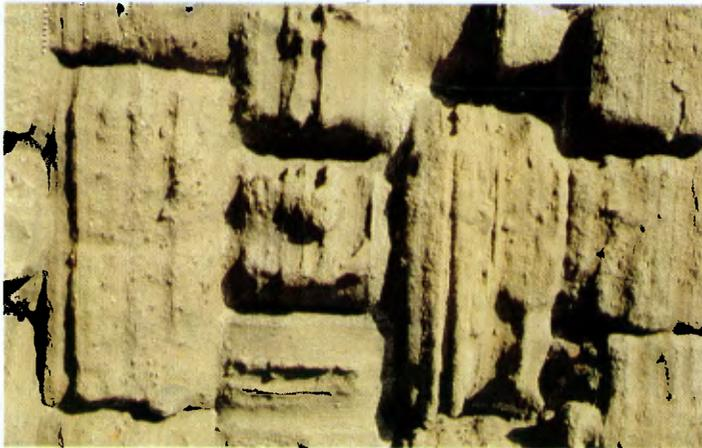
**Figure 6.6** Basement walls of the Tabularium. It is an "opus quadratum" of Pietra Gabina blocks. The texture of this material renders it susceptible to de-cohesion and differential erosion phenomena.
