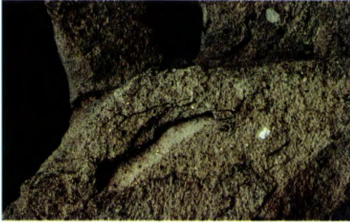
**Figure 6.5** Scaling and alteration on the surface of the Peperino blocks of the podium of the Temple of Antoninus and Faustina. They affect a thickness of only a few centimetres and are more marked at the contact surface between blocks.
