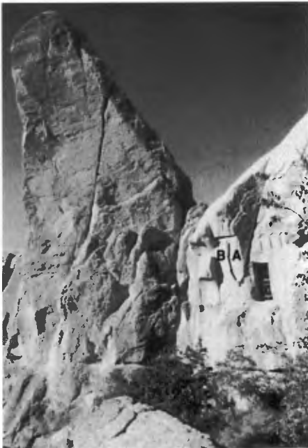
Figure 1. General view of the rear side of Elmalı church indicating potentially unstable rock wedges.
