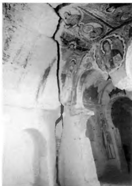
Figure 4. View of the church of Meryemana showing very large open cracks. The dangerous effect of water flow on the paintings can be clearly observed.
