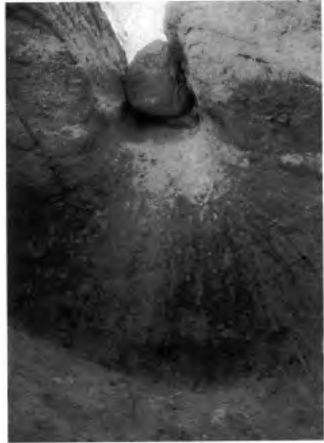
Figure 5. Erosion effect of water flow at the rear side of Elmalı church.
