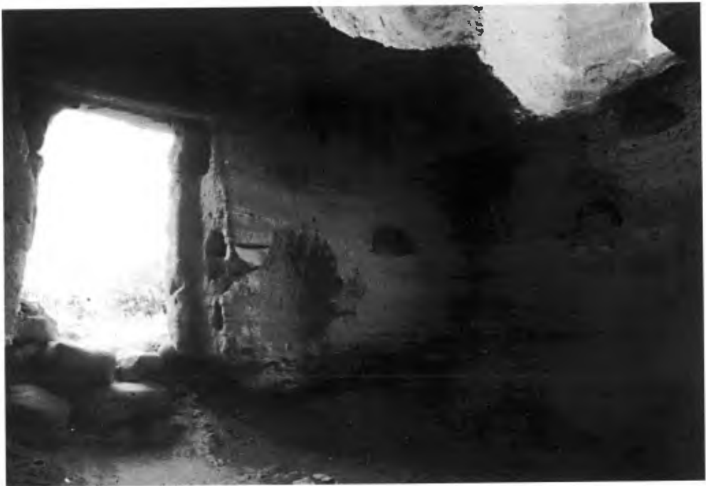
Figure 6. Effects of water erosion at the base of a wall of El Nazar church.
