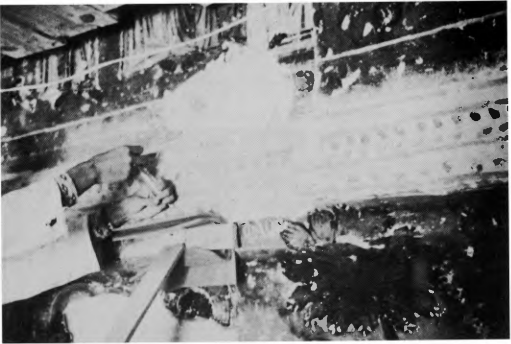
Figure 6. Tokalı Kilise, reattachment of loose plaster.
