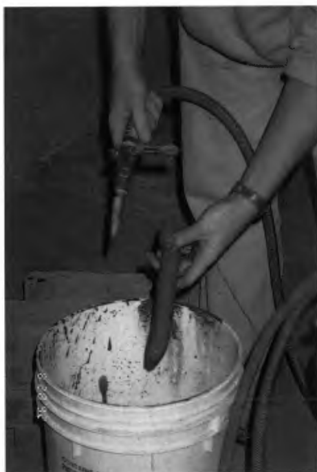
Figures 6-7-8-9. Sequence (clockwise from upper left) taken over ten seconds showing pressure vessel for grout, then the inflation of an anchor and its removal from the injection nozzle.
