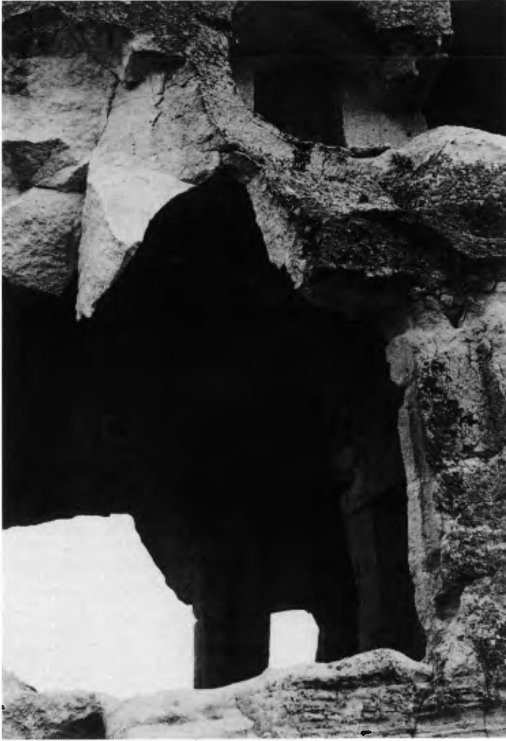
Figure 4. A detail from the entrance to the El Nazar church, showing the overhanging western vault after the fall of the wall in that direction.
