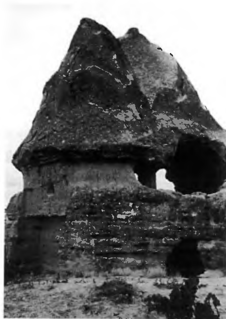
Figure 8. Effects of surface erosion on the soft intermediate layer of El Nazar.
