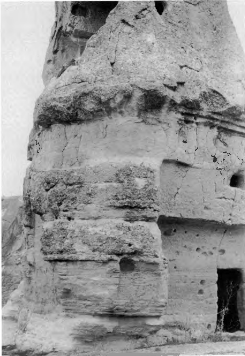
Figure 2. A detail from the southwest corner of El Nazar, showing cracks and eroded areas.
