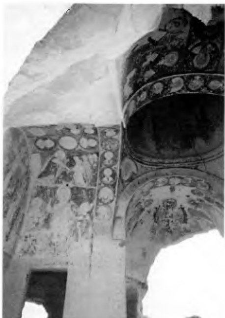
Figure 3. View of the vault of El Nazar where small rock wedges collapsed recently.
