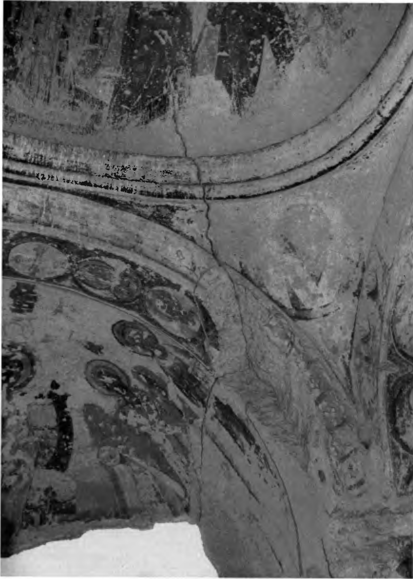
Figure 3. Detail from the eastern vault and dome, with several cracks.
