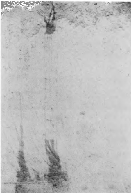
Plate 5. Huaca del Dragón, Trujillo (Peru). Capping of walls with mud mixed with polyvinyl acetate emulsion, resulting in perhaps too hard a surface and excessively smooth. Deterioration of original mudbrick takes place at junction of treated and untreated surfaces.
