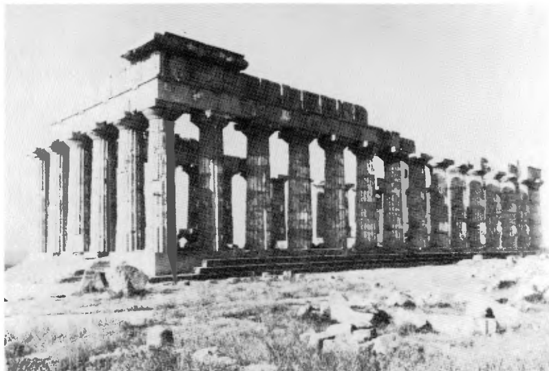
Figure 22. Selinunte, Temple of Hera. Original building elements embedded in reinforced concrete. Considerable errors, which can no longer be corrected, in the reconstruction from a scientific point of view, and dubious aesthetic decisions: an early Classical Greek temple has been partially destroyed through reconstruction.
