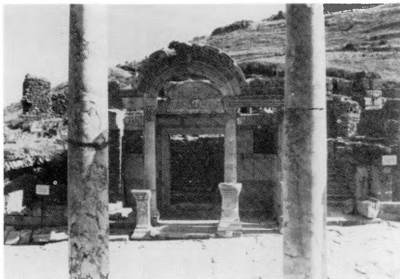
Figure 5. Ephesus, Temple of Hadrian. Anastylis carried out almost exclusively with original building elements.
