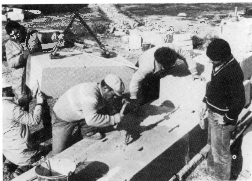
Figure 19. Metapontum, theatre. Natural stone used in rebuilding the outer wall, with strict adherence to ancient technique of working.
