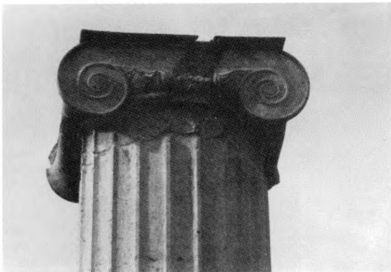
Figure 18. Pella, Greece. Completion of column with natural stone.
