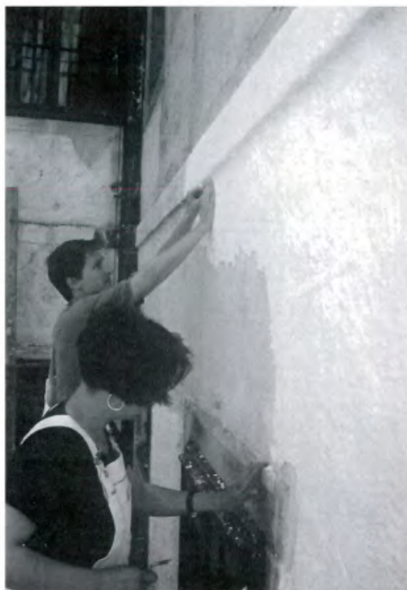
Figure 14. Forchtenstein / Burgenland, castle, main court, facade painting 1687, east facade. Removal of the last desalting compress after treatment with ammonium carbonate and ammonium bicarbonate. Photo: Hammer 1993.
