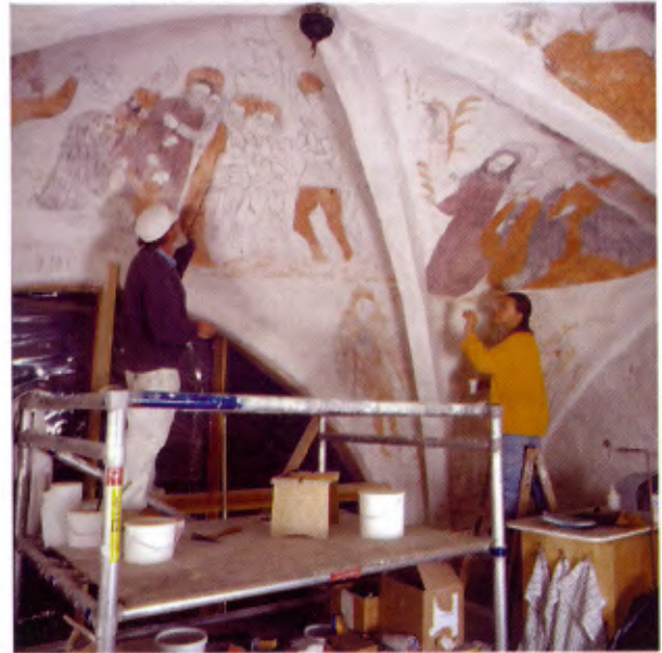
Figure 10. Repairing with lime mortar in Aagerup church. Photo: K. Trampedach
