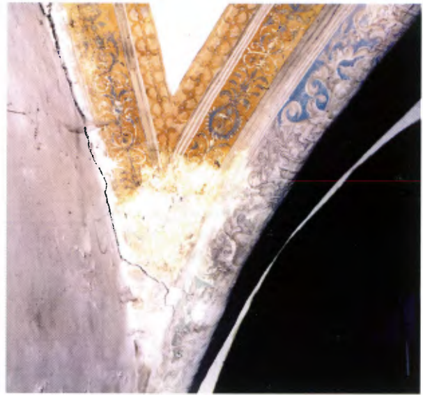
Figure 3. Church of Santa Maria, Villeneuve. The lower parts of arches and vaults suffered extensive water infiltration. The various types of paint layer losses discussed in the text can be seen.
