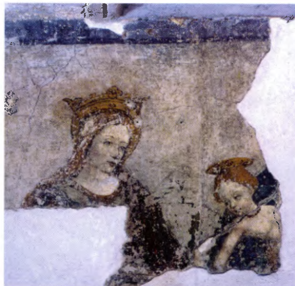
Figure 8. San Grato Chapel, Aosta. Paintings on the façade. Same view after cleaning. The plaster losses are here integrated 2 mm under level with lime mortar.
