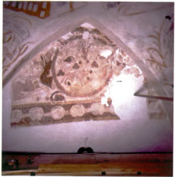
Figure 4. Agerup church. Nave, northern wall. 14th century. During restoration. Limewashing of repairs. Photo: Roberto Fortuna
