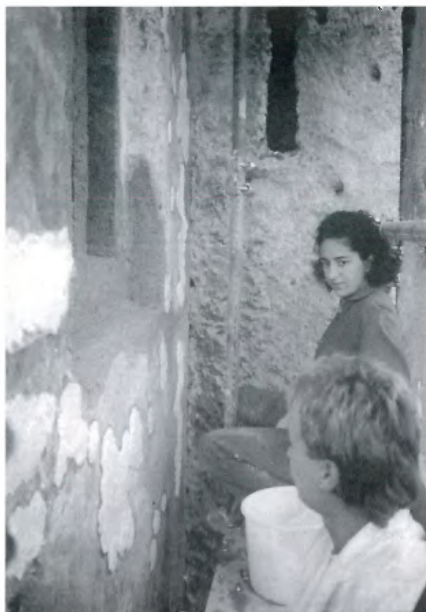
Figure 13. Weissenkirchen, Lower Austria, parochial church, tower dating from the 14th century with original rendering. Cleaning with poultices containing ammonium carbonate. Photo: Hammer 1989.
