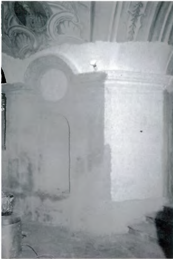
Figure 8. Dürnstein, Lower Austria, former monastery church, crypt, Stucco work and mural painting 17th/18th c. Desalting poultices consisting of different structures: beech cellulose pulps partly stabilized with lime rendering with thin Japanese paper as intermediate layer; lime rendering with polyamide sheet as intermediate layer; note the hygroscopic stains on the compress rendering. Photo: Hammer 1986.
