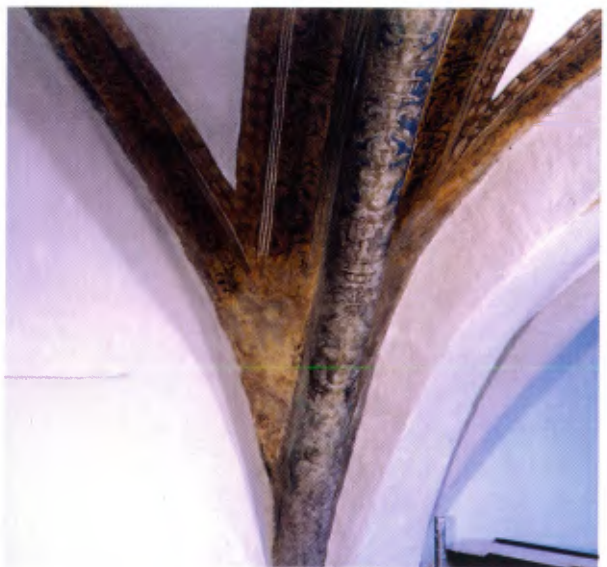
Figure 4. Same view as 3, after restoration. The integration of the brown background frieze has been carried out without any attempt to reconstruct the free-hand painted scrolls. In contrast, the pattern-based decoration of the arch permitted completion of lacking elements with flush filling and 'tratteggio' technique.
