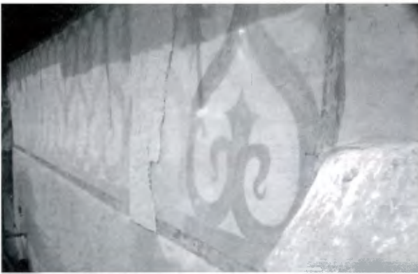
Figure 11. Grades / Kärnten, filial church, 15th century, south facade, detail. A thunderstorm caused considerable infiltration of water. The recently restored facade painting was stained by hygroscopic salts. The stains were removed by a compress rendering put on for a weekend. Photo: Hammer 1987.
