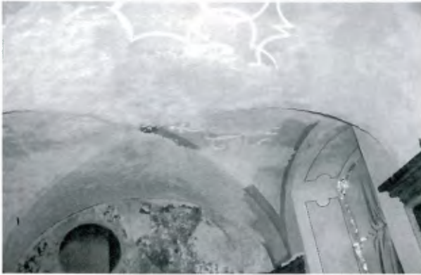
Figure 10. Dürnstein, Lower Austria, former monastery, cloister, vault. Lime stucco work contaminated with soluble salts. Removal of soluble salts by means of lime mortar. A recent glue paint served as a protecting and separating layer. Photo: Hammer 1987.
