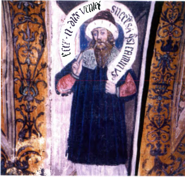
Figure 2. Church of Santa Maria, Villeneuve. One of the prophets (Malachi) on the arch band: note the powdering paint layer and, on the sides, the complete loss of the frieze's paint layer where water infiltration occurred.
