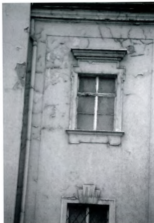
Figure 2. Vienna, Scottish Church, south facade, detail. Because of a blocked drainpipe, salts have concentrated in this area. The paint (ca. 1985) was not permeable to water in liquid form. Salts crystallized behind the paint and caused irreversible damage to the rendering. Decay was increased by thermal dilation of the paint containing artificial resin. Photo: Hammer, ca. 1985.
