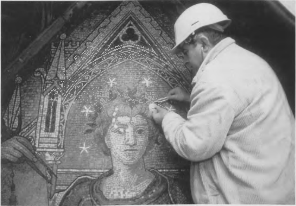
Fig. 6: Giovanni Cucco surveying the mosaic depicting Architecture which is on the north gable. A tuning fork and stethoscope are used to locate the areas of detachment (photo by English Heritage).
