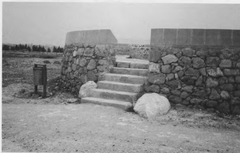
Fig. 5: One of several newly constructed observation points.
