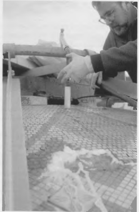
Fig. 2: Injection grouting to re-adhere delaminated surface (photo by Anne Oliver).
