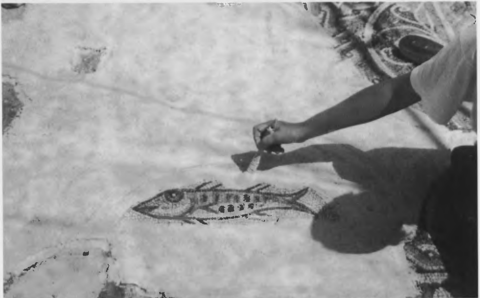
Fig. 5: Consolidation between the tesserae. This operation was carried out by applying a liquid, lime-based mortar.
