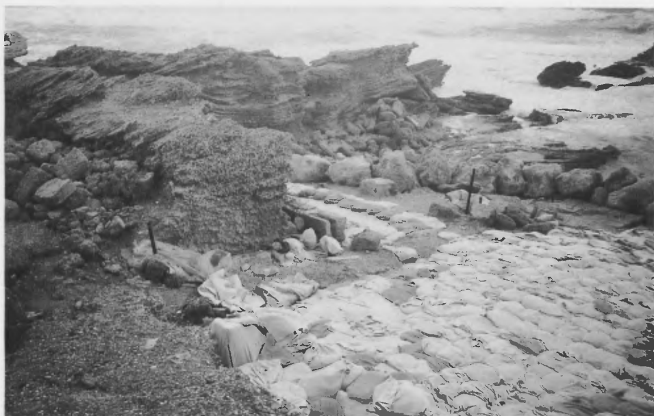
Fig. 2: The site after covering.
