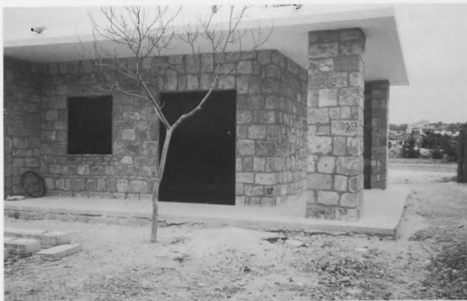
Fig. 2: The new ticket office under construction.
