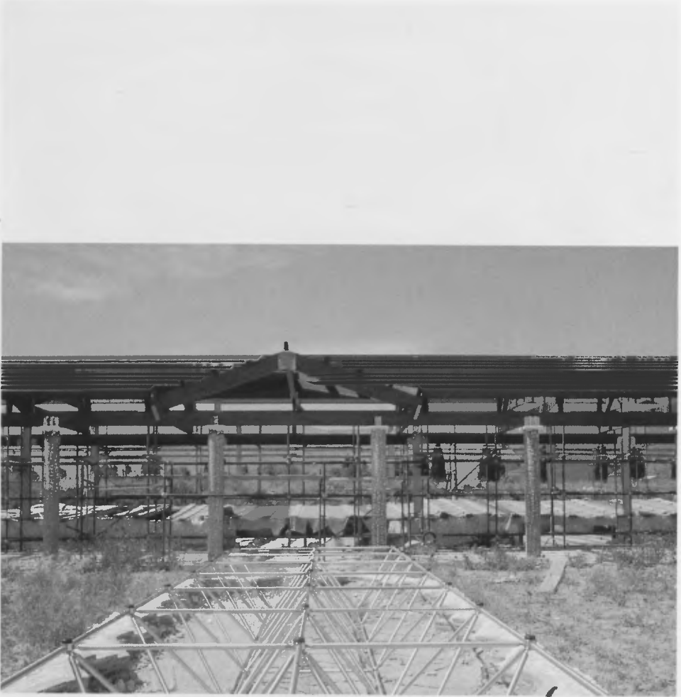
Fig. 6: Corfinio, Augustan domus, construction of the shelter.
