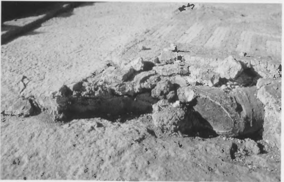
Fig. 6: Tablinum. New bulbous root growth at left edge of cut root section which has caused further damage to raised area of tessellatum and cracking of temporary mortar edging repairs.
