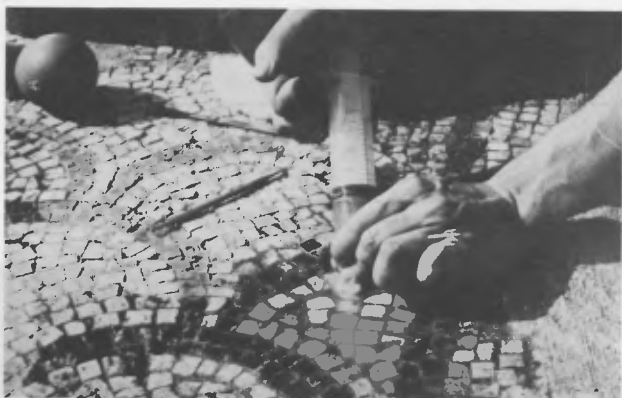
Injection of a hydraulic lime grouting mixture in a floor mosaic at Ostia Antica.
