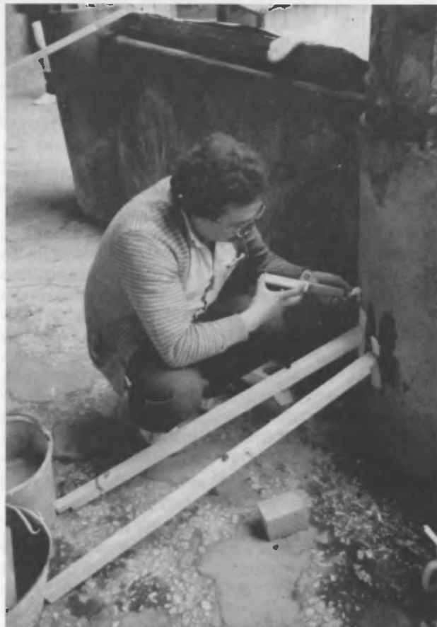
Pompeii. A conservator on the local maintenance staff tries out the ICCROM mixture for the consolidation of painted plaster.
