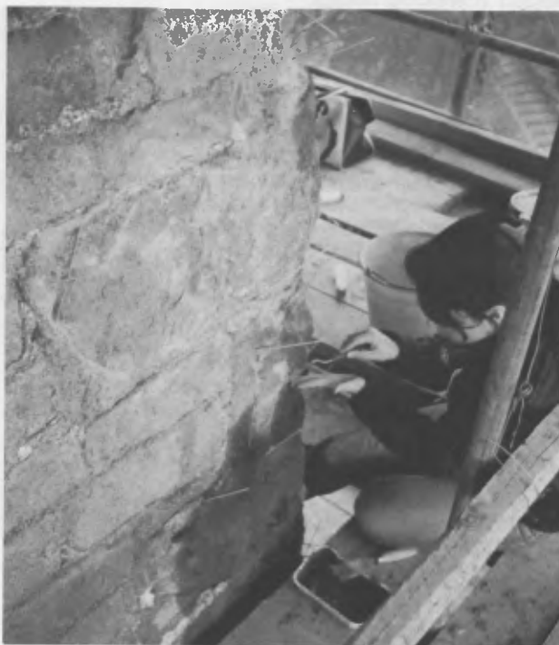
A conservator sealing off an area of wall to be consolidated. Thin sticks are inserted to provide holes for injecting hydraulic grout.
