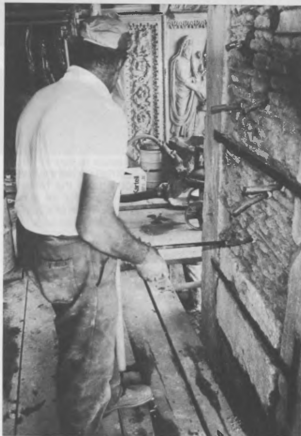
Rome: Arco degli Argentari. Holes were drilled up to 1.20 m deep into the sides of the weakened pier, seen here from the back. After the structure was dampened, a grouting mixture was injected from the bottom up.
