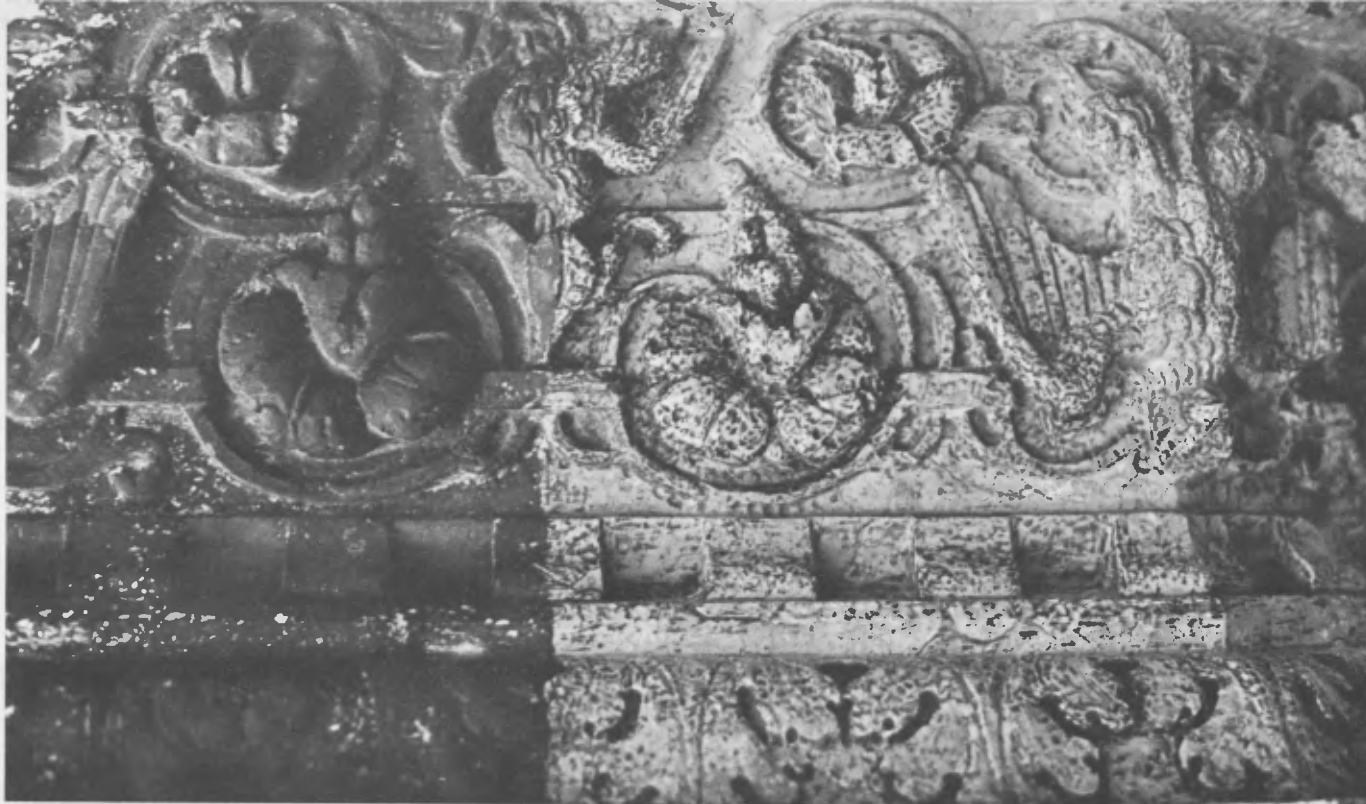
San Petronio in Bologna: detail showing partly cleaned frieze using sepiolite method.
