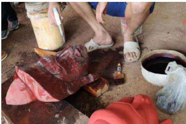
Fig 35e. Multiple application of chemical solution and cleaning
