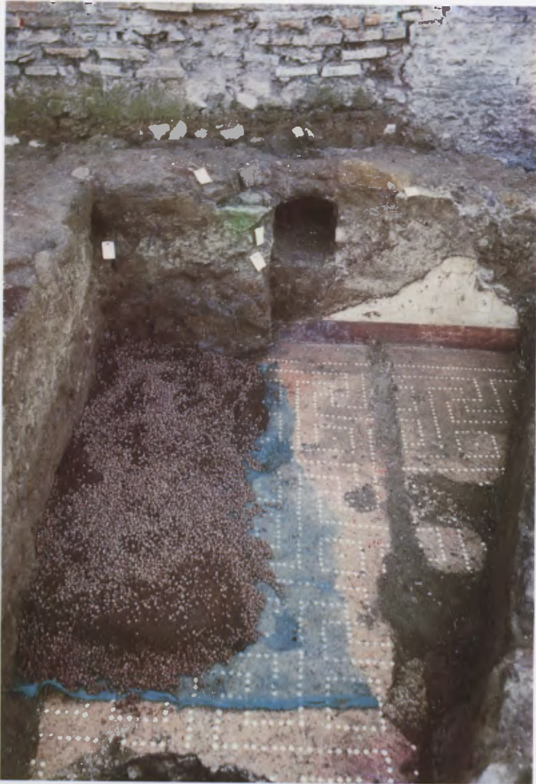
Back-filling of the pavement using plastic net, expanded clay mixed with pozzolana.
