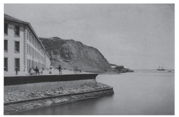
Figure 5. Coastal border and customs' warehouses, Las Habas in the west of the city. Clearing and levelling work was conducted on Artilleria hill to generate surface area for customs and dock-related activities.
