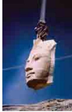
Abu Simbel, Egypt. Dismantling the Temple of Ramses II by means of a derrick crane. © UNESCO/Nenadovic
