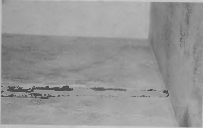
Signs of mould (dark areas) on the interior of a fire-proof safe.
