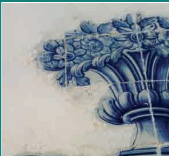
FIGURE 3 Salt efflorescence at the edge of a panel.
