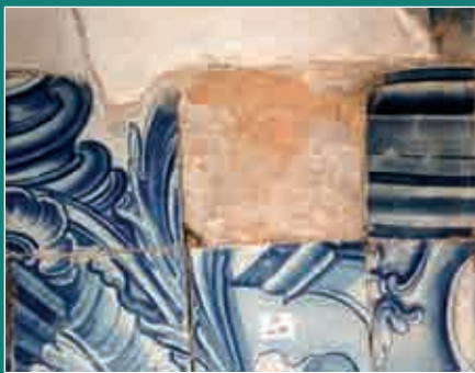
FIGURE 9 a, b, c Filling of a large gap with a replica tile.
