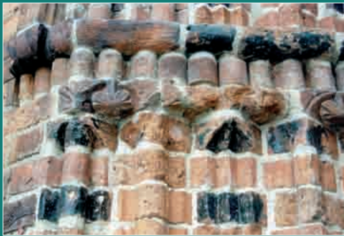
FIGURE 5 (LEFT BOTTOM) Extremely damaged bricks of the St. Jakobi church in Perleberg, Brandenburg, Germany.
