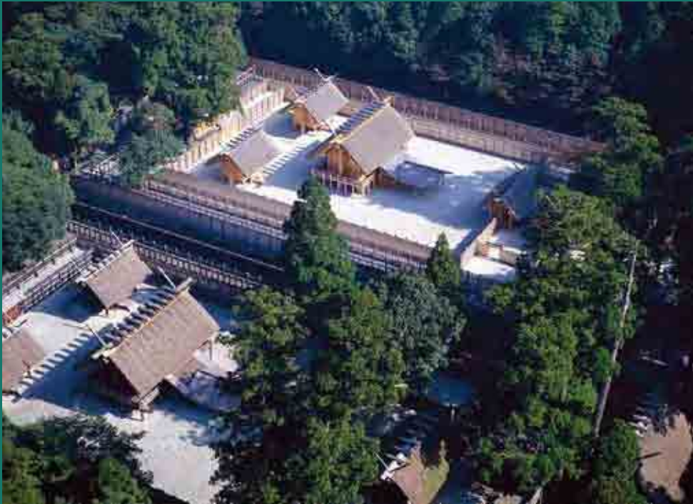
FIG. 7. Ise Shrine Inner Compound. Aerial photo showing new and old buildings during the reconstruction transition period; the older compound will be dismantled after the transition ceremony (photo Jingu Shicho)
