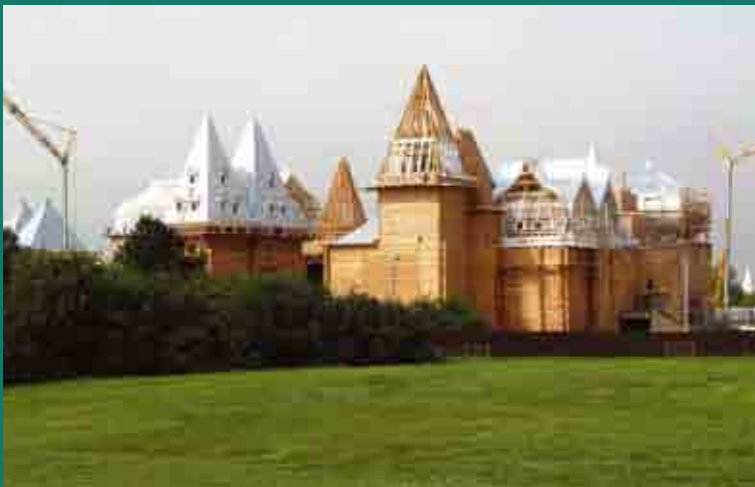
FIG. 10. The Palace of the Tsar Alexei Michailovitch in Kolomenskoe, Moscow, Russia, a wooden 17th-century structure dismantled in the second half of the 18 th century and currently being re-erected with a concrete skeleton and wooden facades (photo Natalia Samover, 2008)
