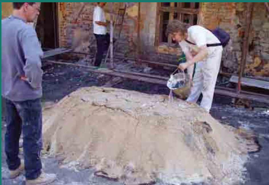
FIG. 4. H. Weissenbach instructing the participants of the 2005 international course in lime slaking (photo author)
