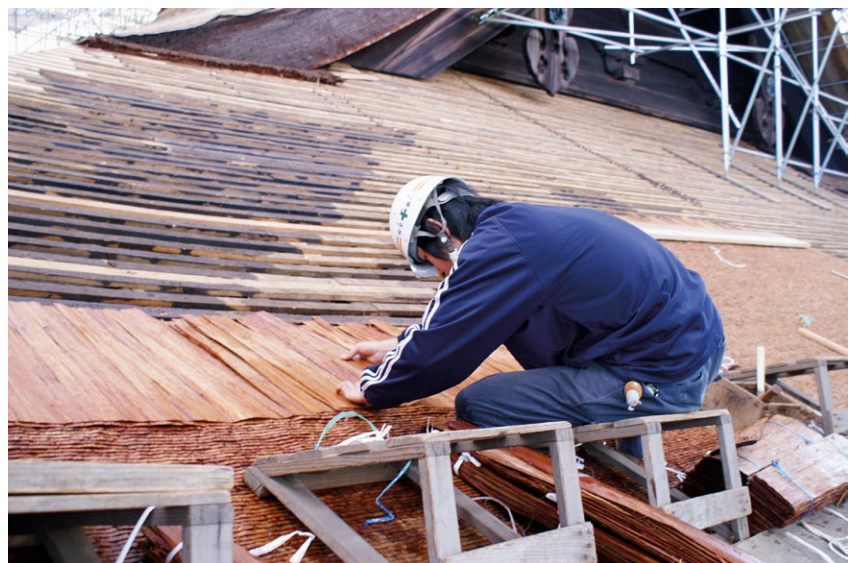
Figure 2 Roofing with cypress bark.
