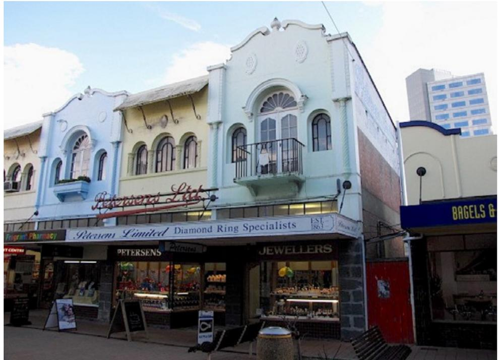
► **Fig. 7.** New Regent Street facades looking west prior to the earthquakes. The concrete beam at first floor level is visible in the end elevation of the row (Source: CCC, August 2010)
