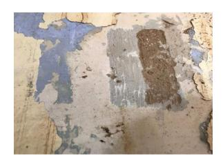
The restoration work allowed us to uncover more about the history of the building and how it was developed. The image on the left shows a test the painted layers of the interiors.
