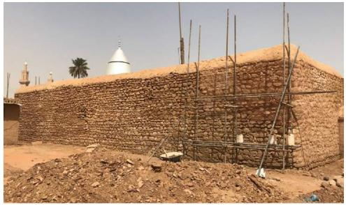
$\label{the:cleaned} This is the stone wall of the Khalifa House.$  We cleaned off the mud and repointed the stone.
