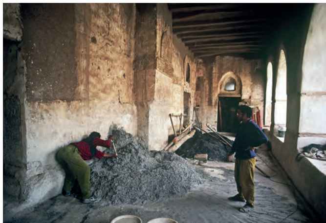
Fig. 2. Preparation of the qudad mix at al-'Amiriya. (Photo by author.)
