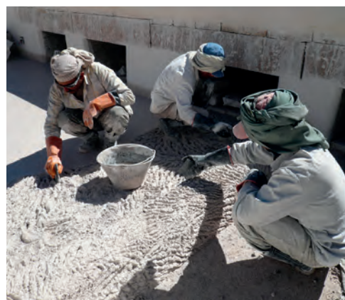
Fig. 3. Pounding the qudad waterproofing on the roof of the new ablution building for the Grand Mosque of Shibam Cocoban, Yemen. (Photo by author.)
