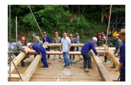
**Fig. 25.** Cooperation in action: carpenter guides work in reassembling a bridge bean frame, Xuezhai Bridge, Taishun County Wenzhou City, Zhenjiang Province, China (Source: Huang Zi)
